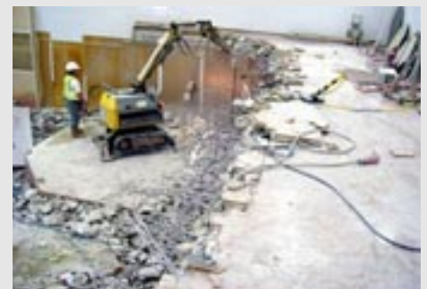
Noiseless removal of mezzanine floor with Brokk robot
