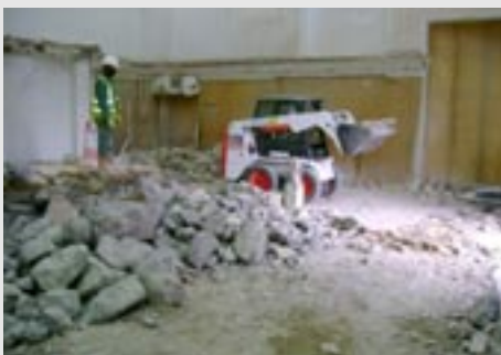
Concrete debris is removed by skid loader to go for recycling.
