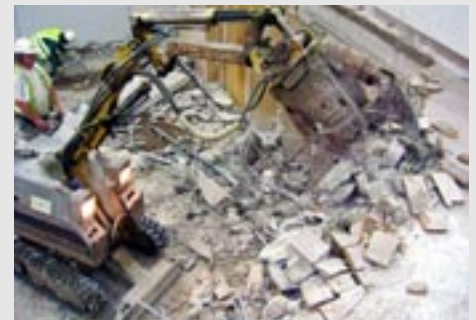
Vibrationless removal of mezzanine floor with hydraulic jaws on robot
