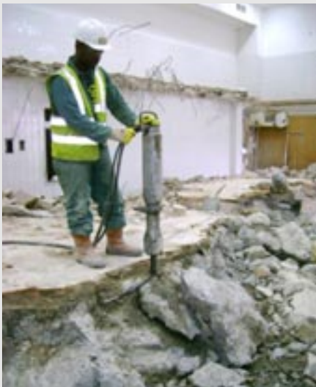
Hydraulic burster cracks up heavily reinforced concrete tank bases without vibration, noise or dust
