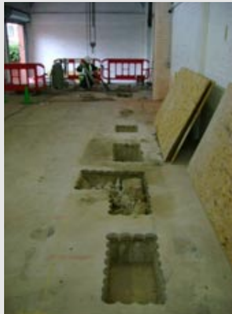
Openings Stitch Diamond drilled in substation floorslab
